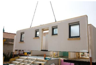
Transforming construction (up to £170m)
